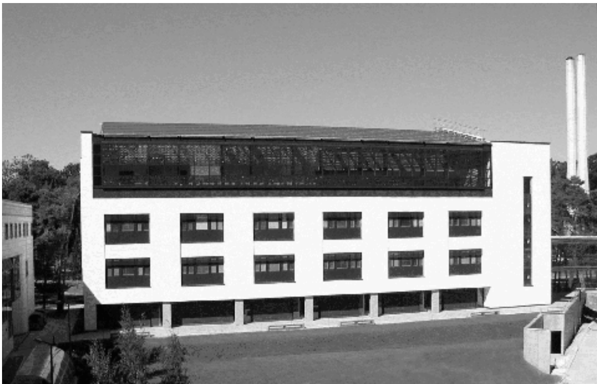
Fig. 10. The ZICER building showing the photovoltaic array on the top floor.
