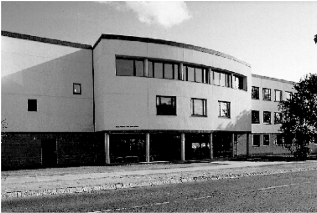
Fig. 8. The Elizabeth Fry Building completed in 1995.
